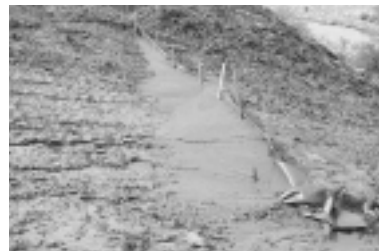
Sediment fences need maintenance to remain effective
