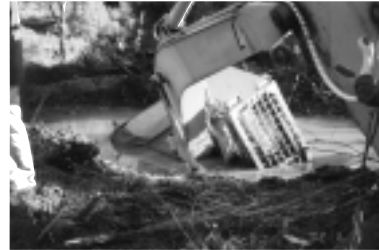
Keep machinery off wet and unstable areas
