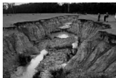
Badly designed drainage works can trigger serious erosion
