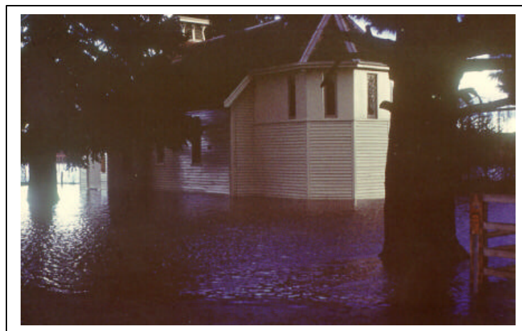
Plate 5: November 1974 – Flooding at the Derwent Church of England at Bushy Park. Floodwaters rose to the base of the doorstep and the top of the sandstone foundations.
