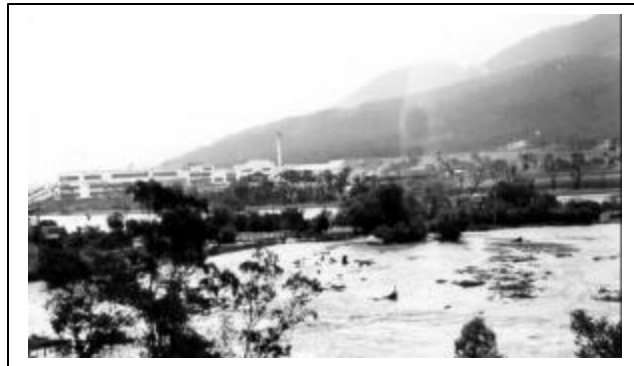
Plate 1: Flooding during 1940 near the Boyer Mill looking from the Molesworth Road across Sorell Creek. The Lyell Highway is in the middle distance.
