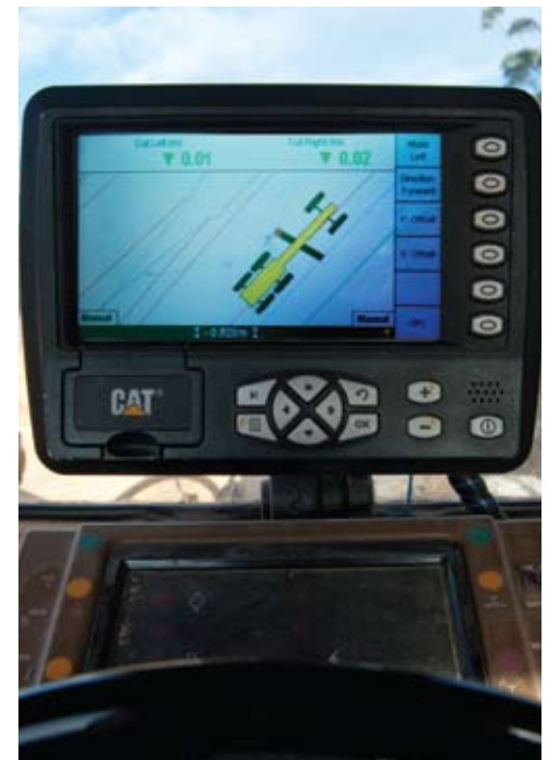
GNSS guided earthmoving equipment used in construction of the Kingston Bypass. >>>
