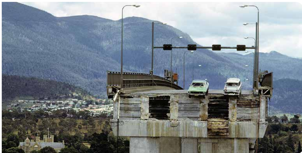
Cars balance on the edge of the collapsed Tasman Bridge, 1975.
